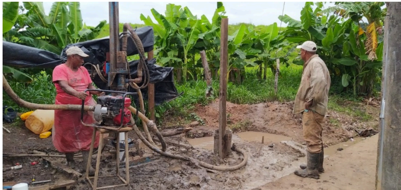
Punta Masaya well drilling, December 2023
