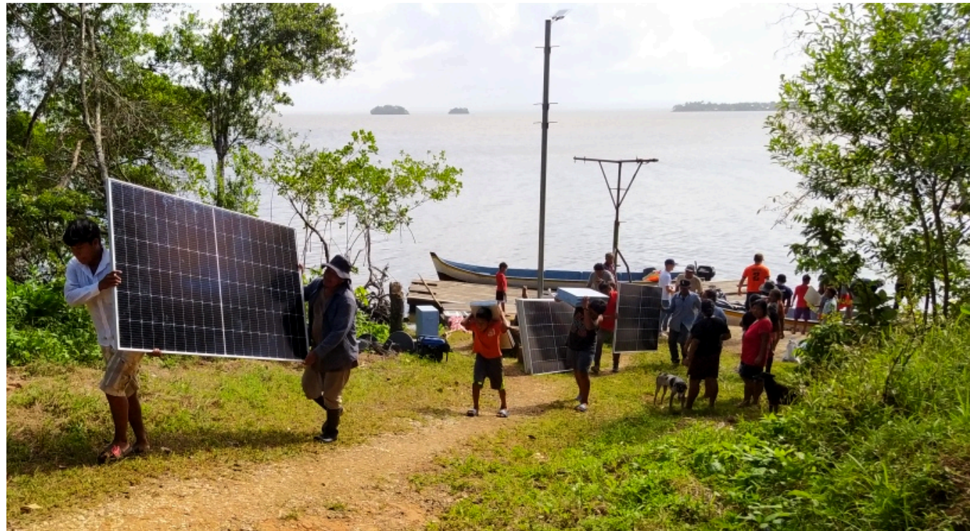
Delivery of equipment to Rama Mainland, December 2023
